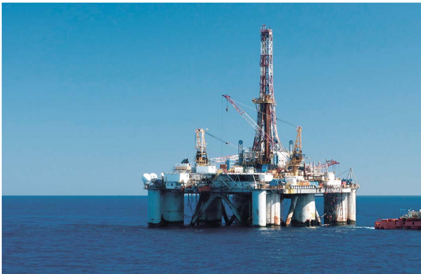
Offshore drilling. Source: Shutterstock.
